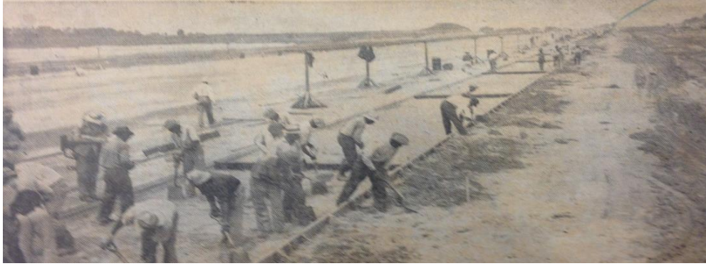
Workmen constructing one of two runways which, when completed, will be approximately two miles long each
