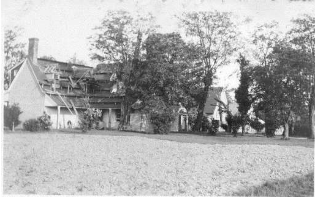
196. Renovating the Mansion, putting shingles on the "New Room". Courtesy of Historic Sotterley
