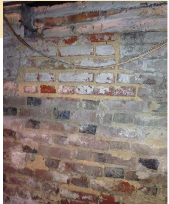
Figure 23 Secret Tunnel Basement Wall Repairs
