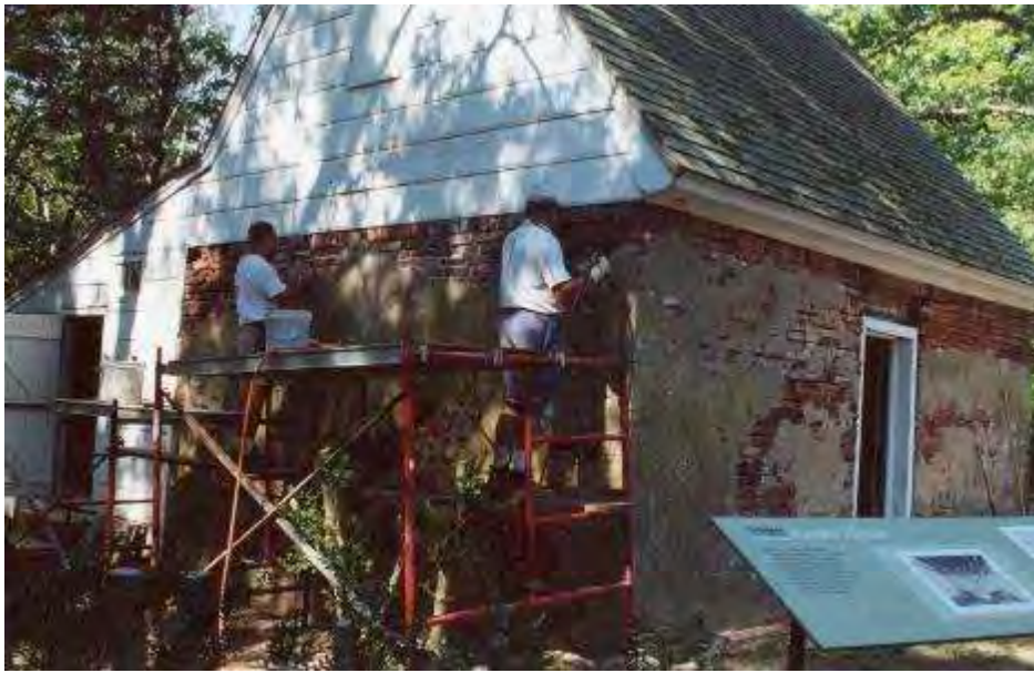
40. The brick walls of the smokehouse being restored. Courtesy of Historic Sotterley
